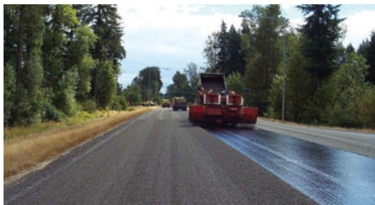
PHOTO: WASHINGTON STATE DEPARTMENT OF TRANSPORTATION
