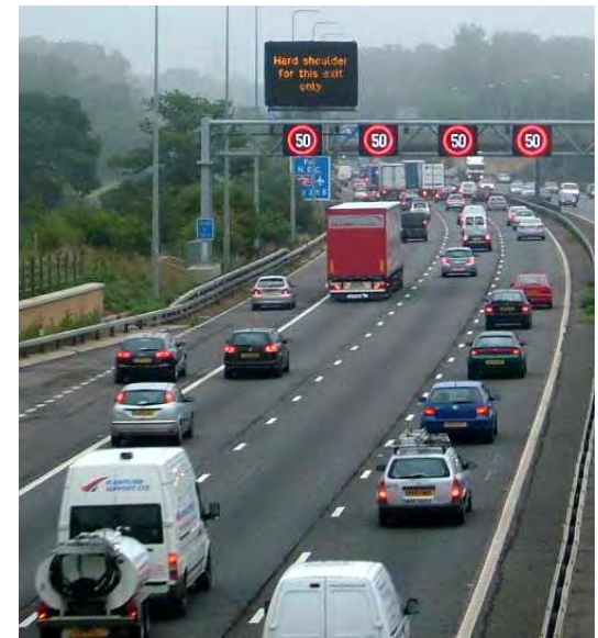
M 42 Speed Harmonization and hard shoulder lane in England. (UK Highways Agency)
